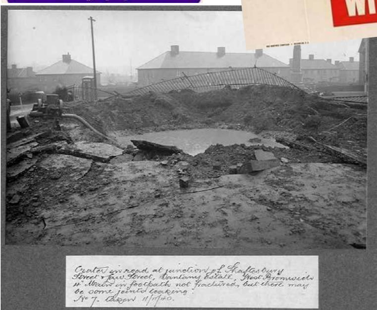
Crater in road, at junction of Shaftesbury Street & New Street, Birmingham, 1941. Footpaths & drains in footpaths not fractured, but there may be some jointed leakings. No 7. 11/1/40.
